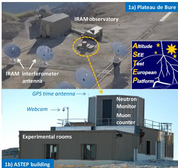
**Fig. 1.** (a) General view of the Plateau de Bure. (b) External view of the ASTEP building showing the new extension (first-floor) designed to host the Plateau de Bure neutron monitor (PdBNM).
