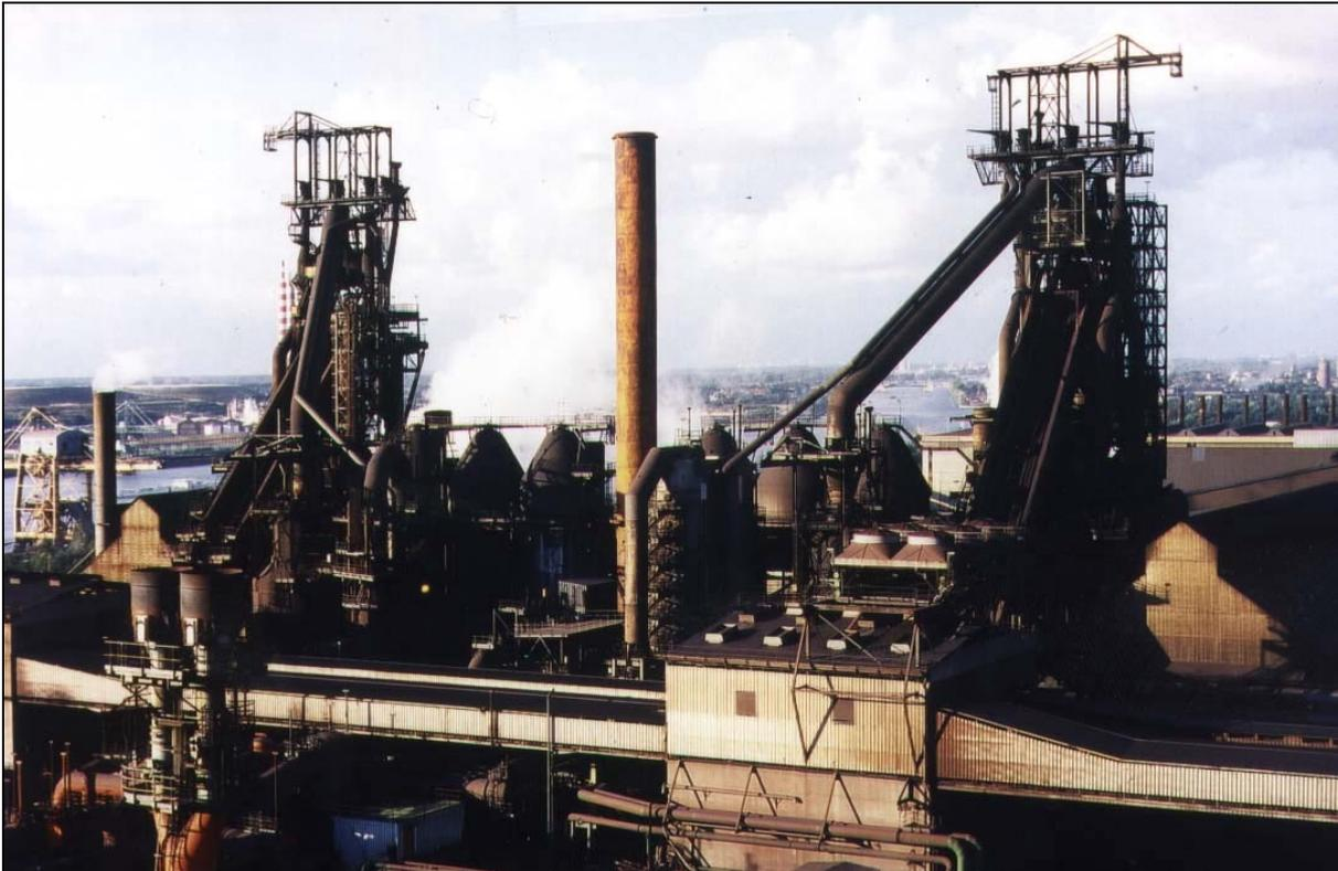
**Figure 7.1 : : General view of two blast furnaces with three hot stoves each and the stack for the waste gas from the hot stoves**
